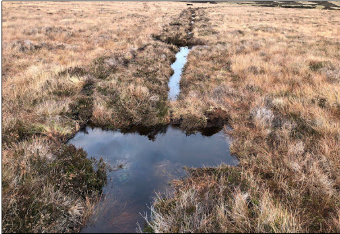
Plate 2-2. Example of peat dams to be used for on-site forestry drain blocking. This will re-establish and maintain a hydrological regime for the required peatland rehabilitation.
